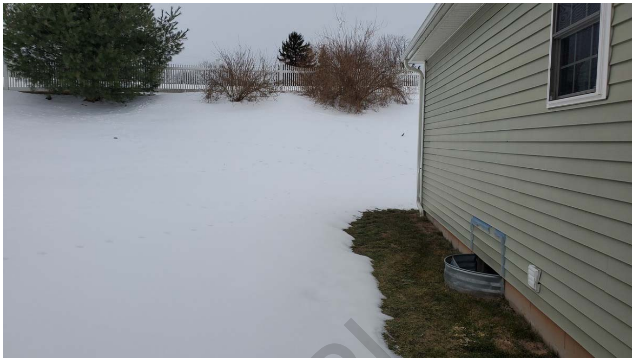
Grade to the west slopes toward structure. Drainage system functionality should be verified.
