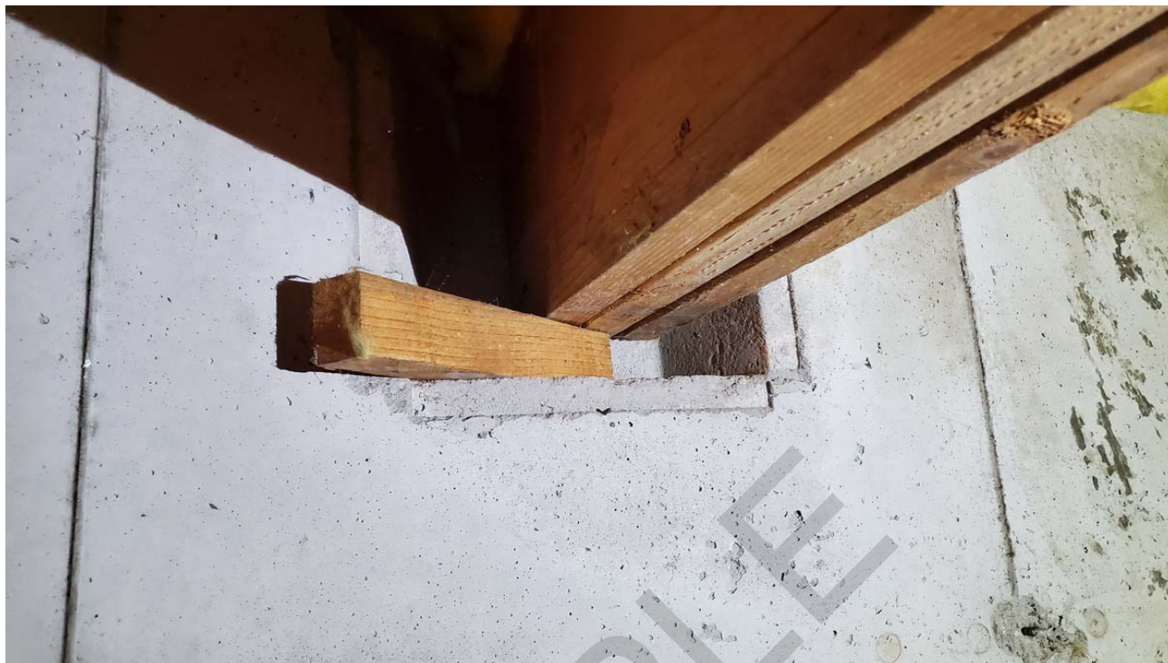
Loose shim at beam pocket, south – western beam.
