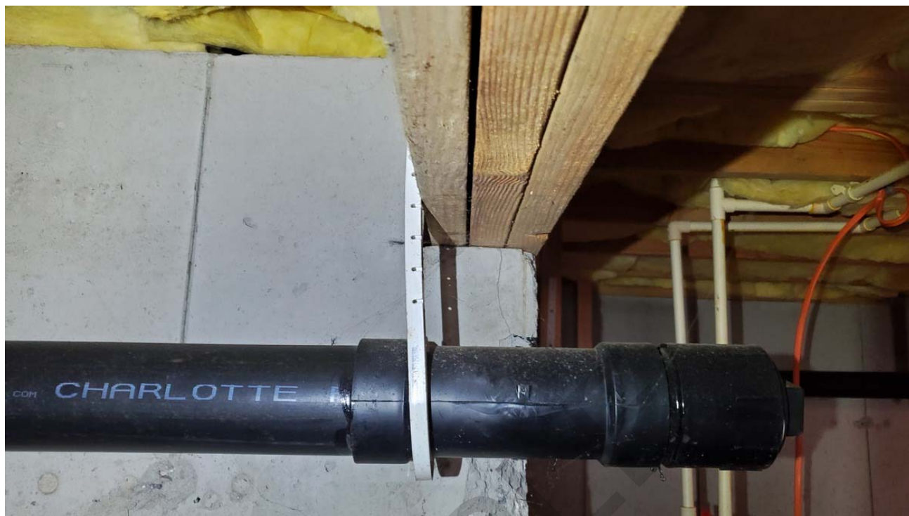
Cracked beam pocket, eastern-most beam.
