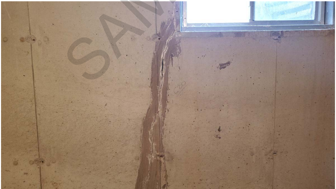
Additional view of prominent crack in foundation south wall.
