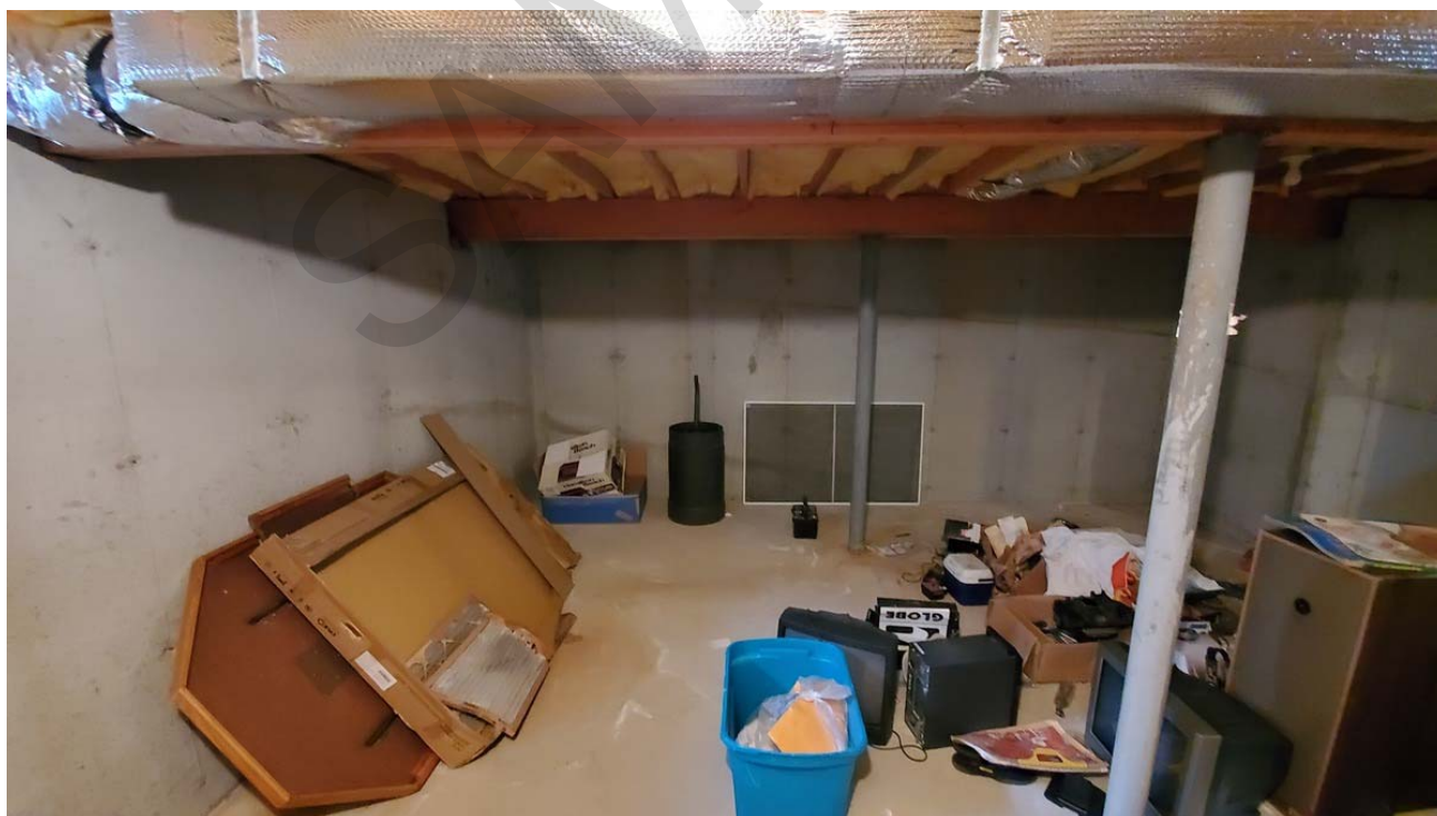
Efflorescence and water stains observed on foundation walls and floor slab.
