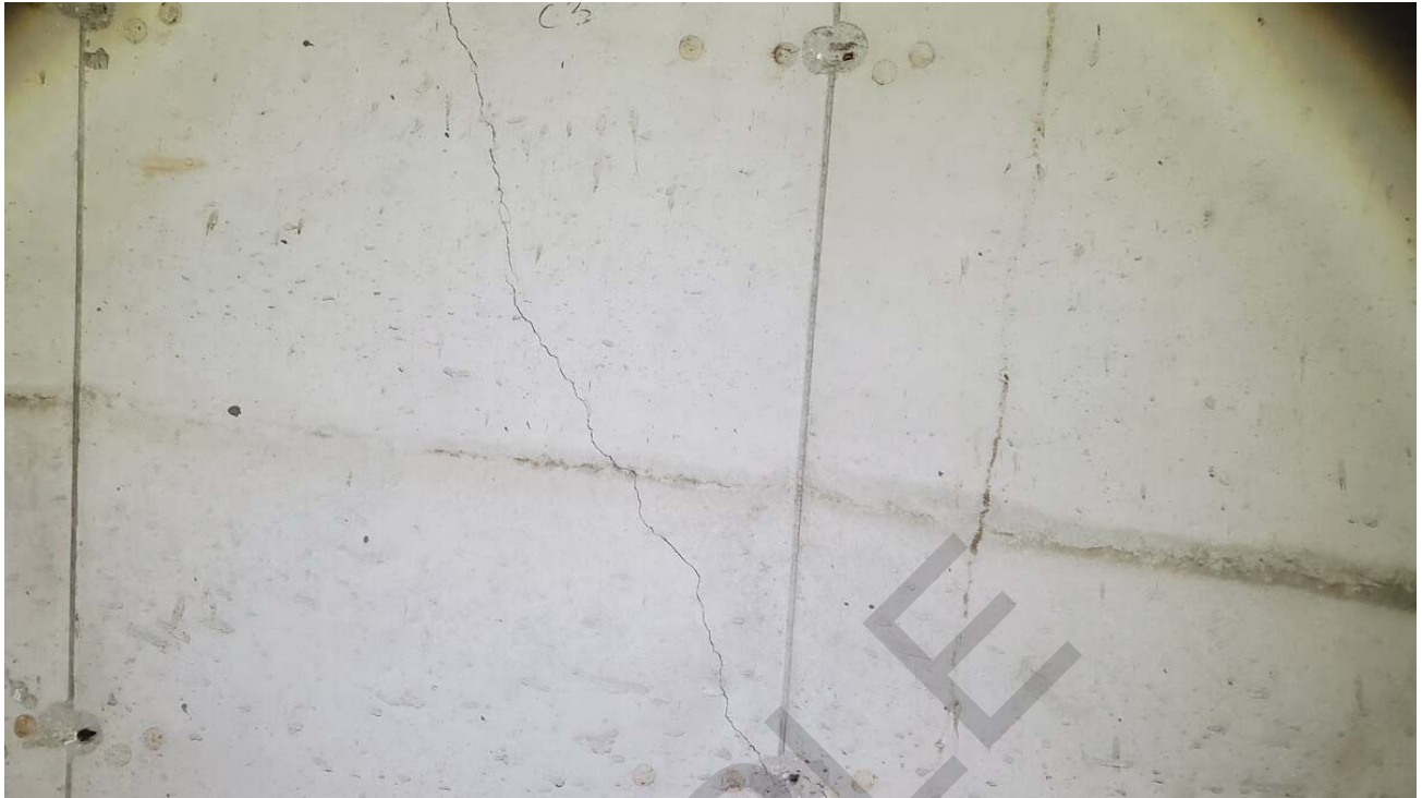
Diagonal crack in foundation west wall.
