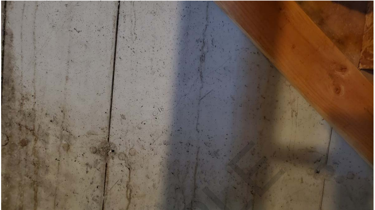
Diagonal crack in foundation east wall.
