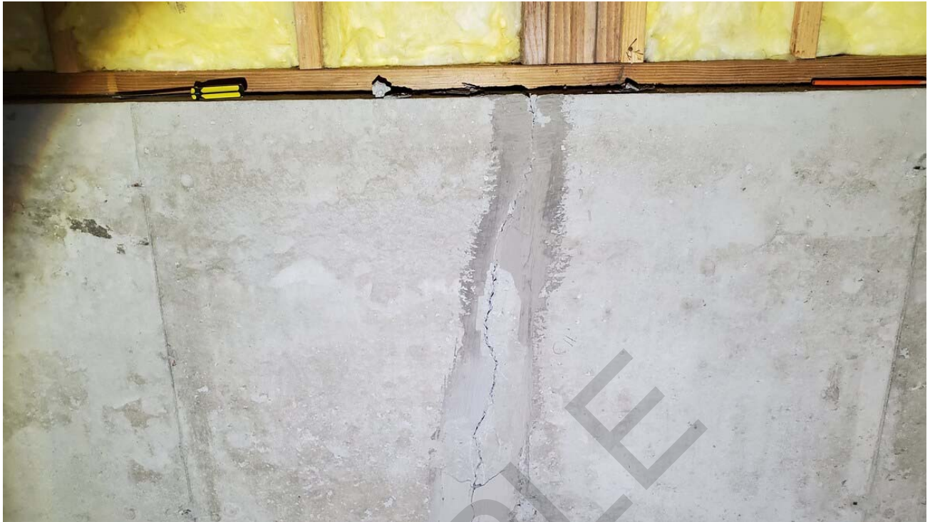
Prominent crack in foundation north wall.
