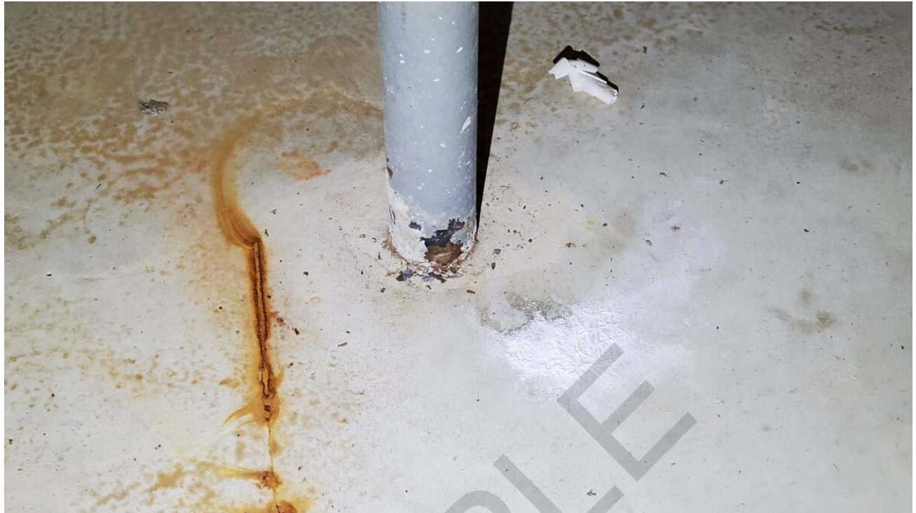
Corrosion at column bases.
