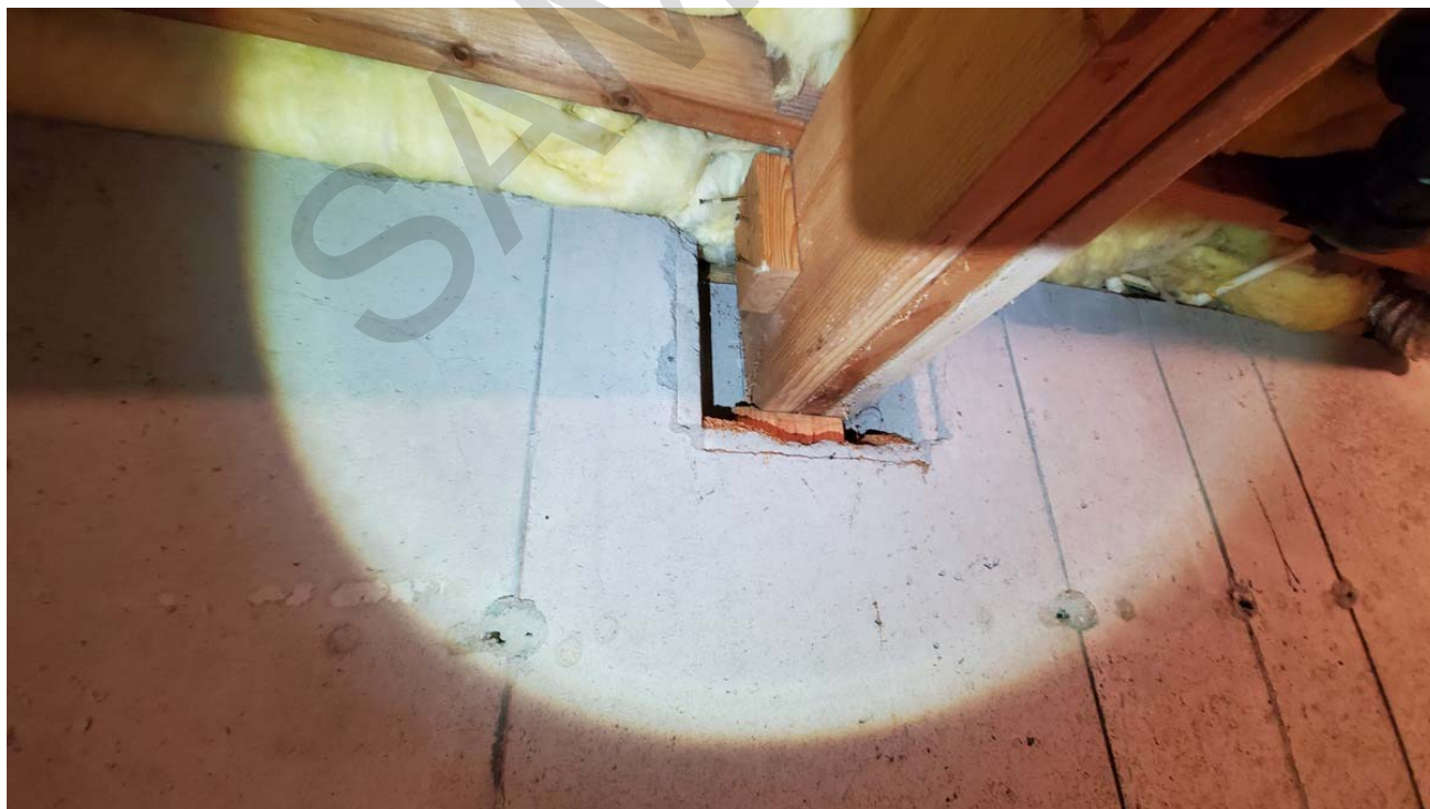
Inadequate bearing provided by shim, beam alongside basement stairway.
