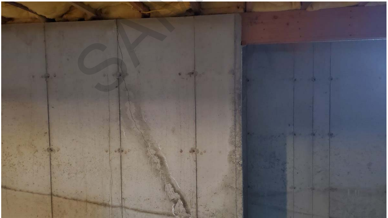
Diagonal crack in foundation west wall, with efflorescence.
