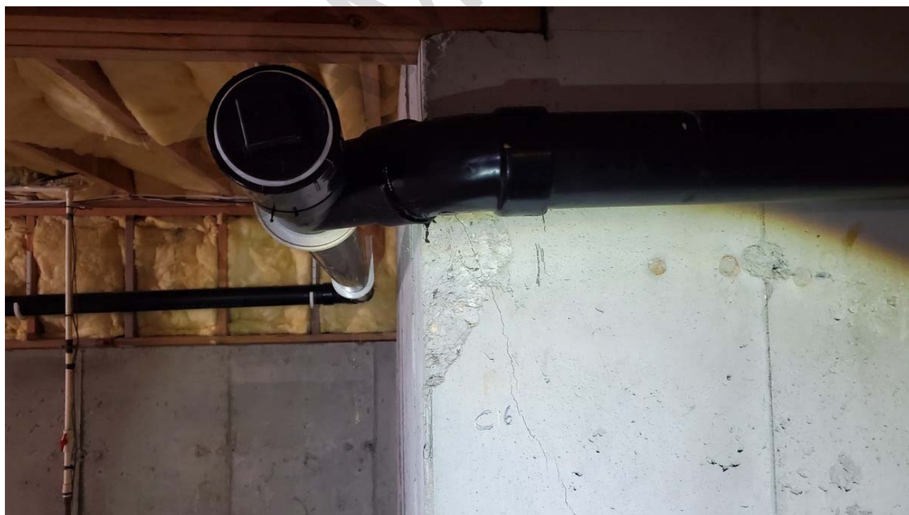
Additional view of crack at beam pocket, eastern-most beam.
