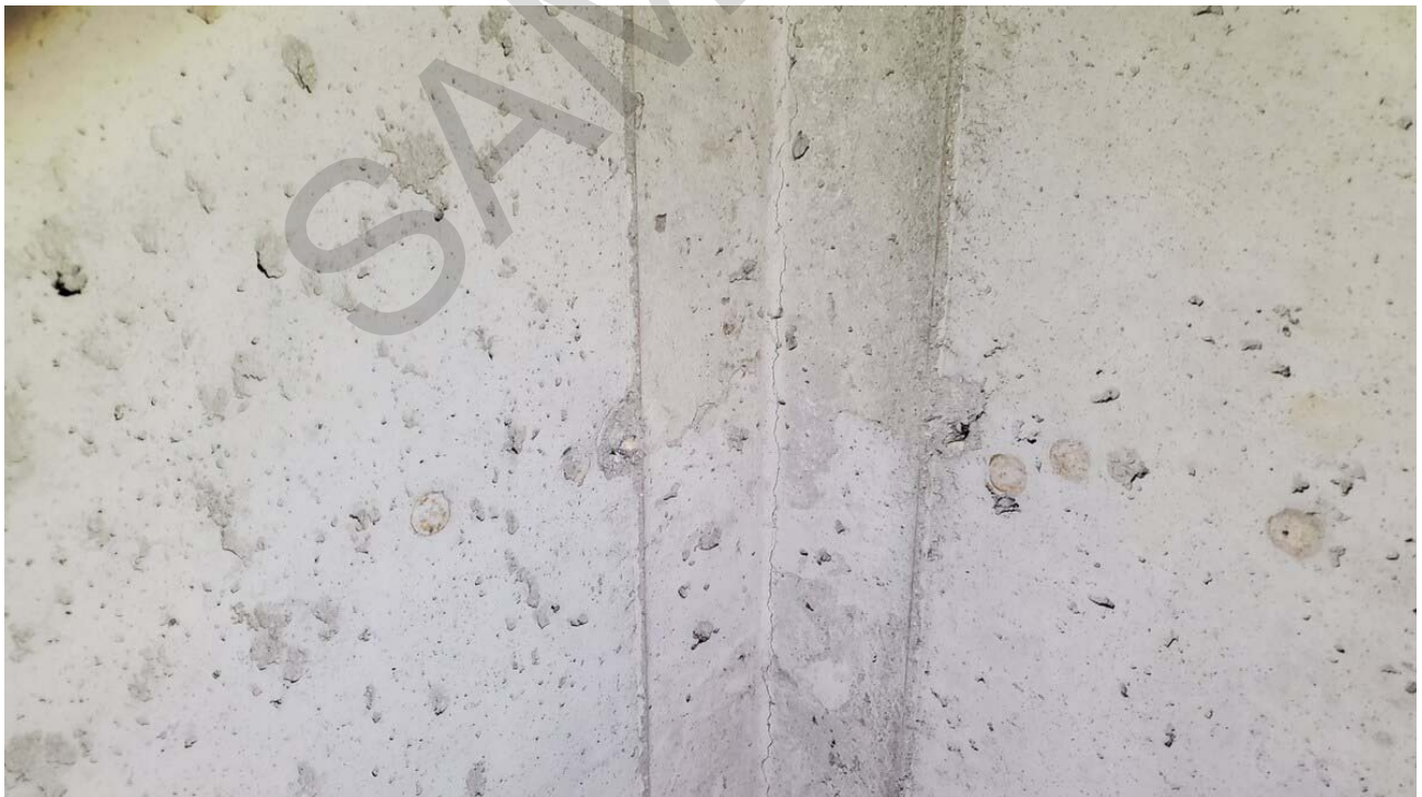
Hairline crack (Typical)
