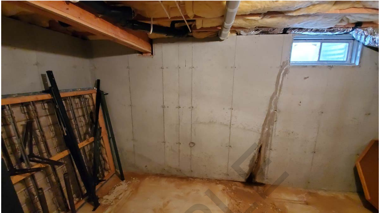
Prominent vertical crack in foundation south wall.
